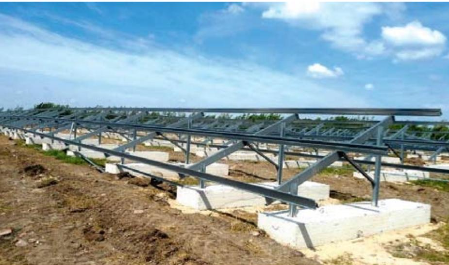
Hill & Smith offers various foundations such as concrete ballast foundations, pile driven foundations and anchor foundations.
