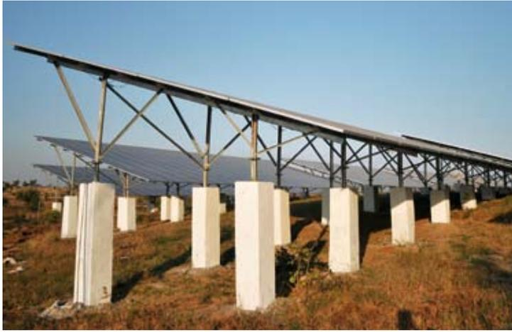
India has drastically varying soil profiles. Nuevosol therefore offers a variety of new foundations such as under reamed piles and rod foundations with chemical grouting.
