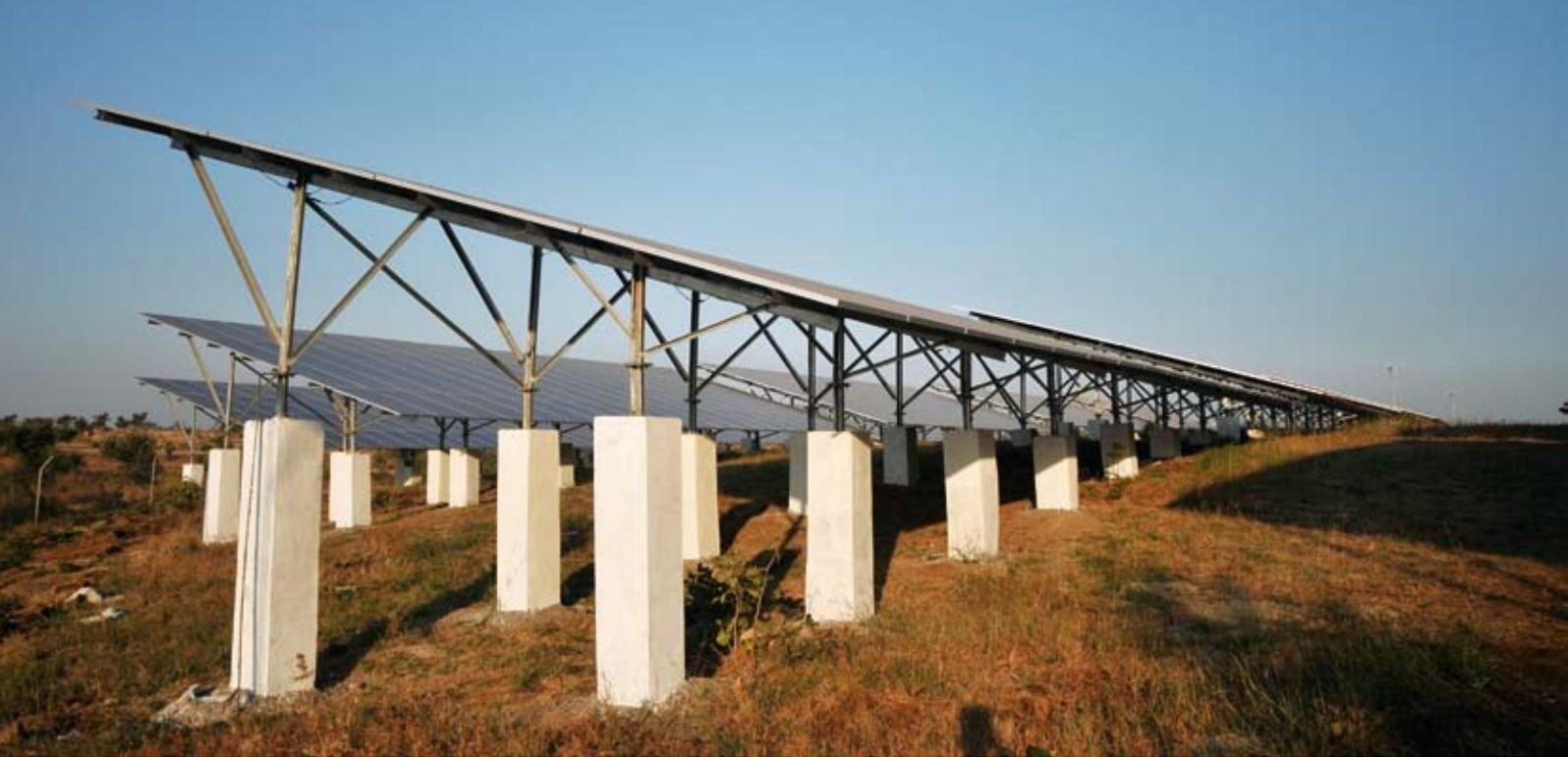
Here a ground-mounted system from Sika is being installed. The back rails are applied to the rear sides of the modules using adhesive technology.
